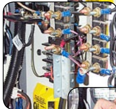
Install plain washer, lock washer, and nut.
